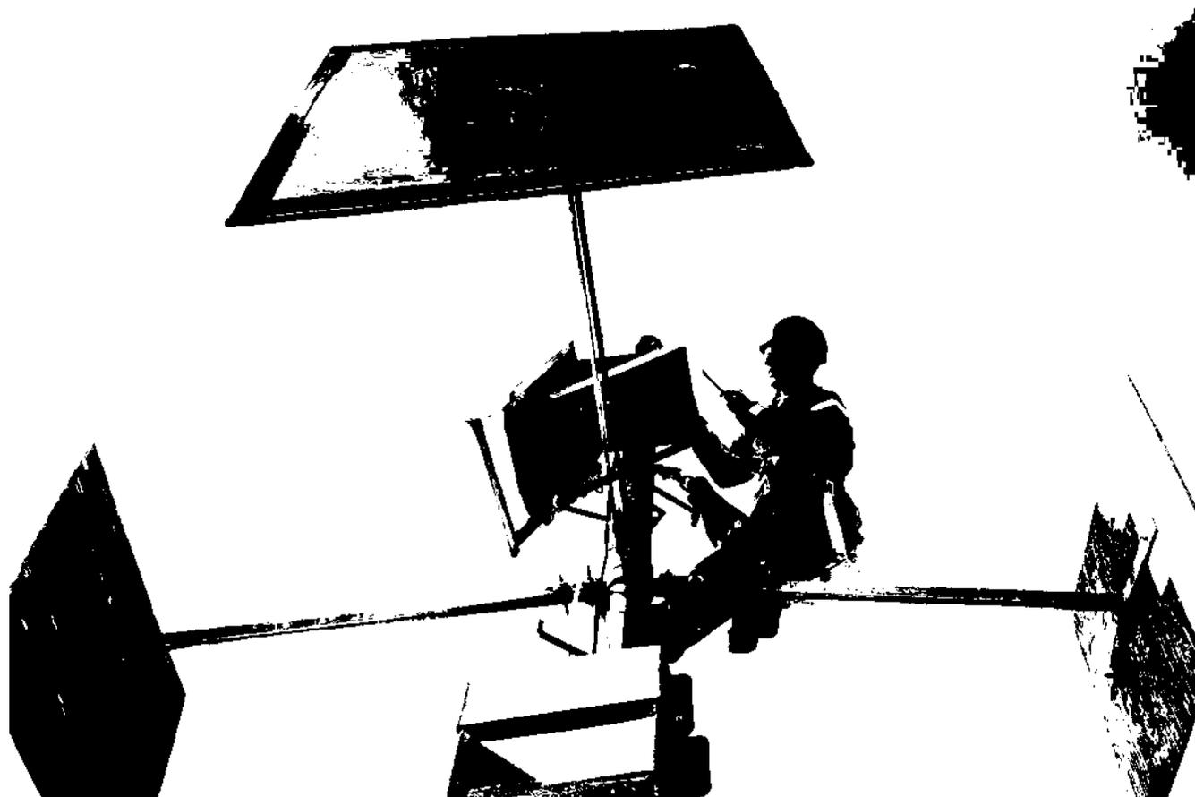
An electrician's mate stationed with Aids to Navigation Team (ANT) Woods Hole, climbs a structure to replace an outdated 155 millimeter lantern with a self-contained LED Carmanah light. ANT Woods Hole is responsible for maintaining 250 buoys, 20 lighthouses, and 54 structures along the coast of southeastern Massachusetts. U.S. Coast Guard photo by Petty Officer 3rd Class Andrew Barresi
